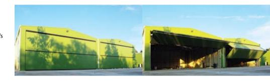
unbraces the gates and they start to rise. Gate rises to the top with the help of lifting straps and the upper end rigidly attached to the upper lintel. When doors reaches the predetermined height of the opening disconnectors on the electromechanical drives stops them.
